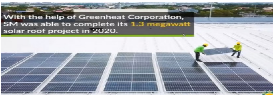
SOLAR ROOFTOP. Photo shows Green Heat Corp. 1.3-megawatt roof-mounted solar power plant at SM City Bacoor in Cavite. The solar power plant can generate 40 percent of SM City Bacoor's 1.6-MW daily power demand. (Screenshot from Green Heat online briefing)
